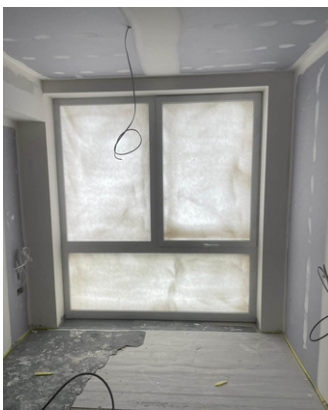
Intelligent Protect install.
