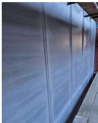
Intelligent Protect install.
