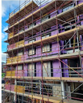
Tower block install.
