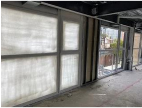
Intelligent Protect install.
