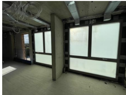
Full temporary protection.
